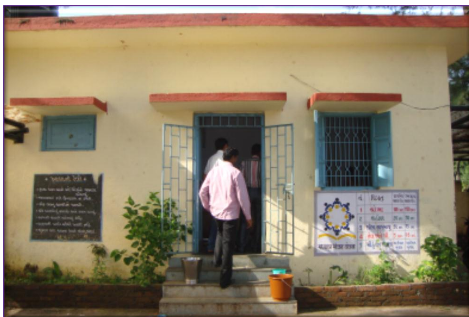
Well maintained kitchen shed at GMS Patlara.
